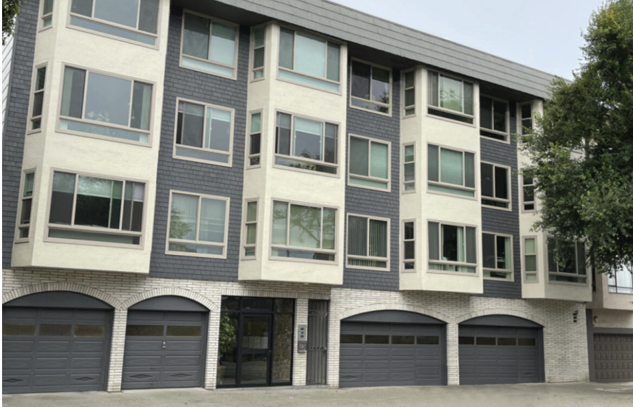
Residential structure with tuck-under parking
